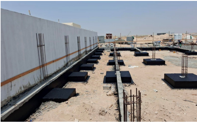
BASES CAST, HOLDING-DOWN BOLTS SET TO SURVEY
