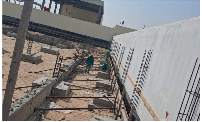
BOUNDARY WALL AND COLUMN STARTER BARS
