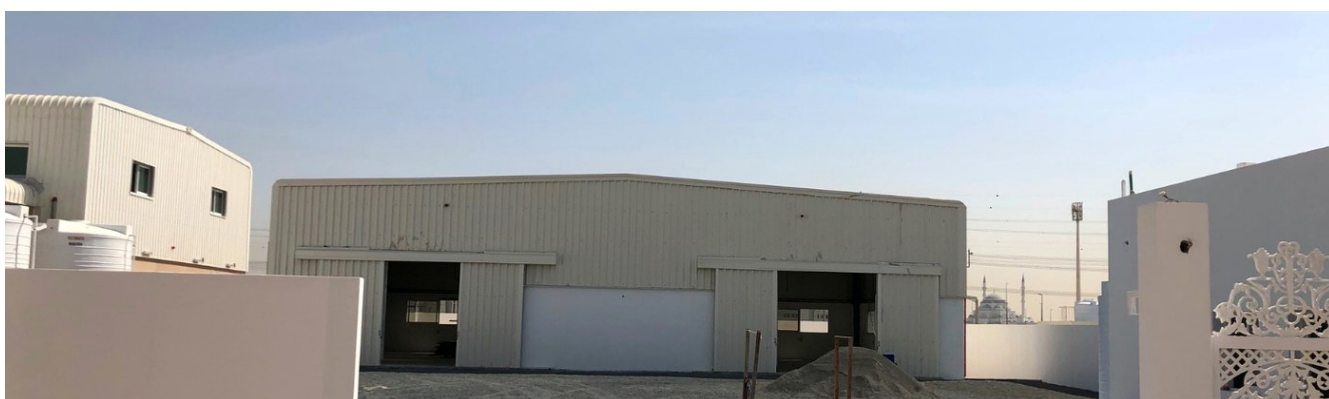
COMPLETED BUILDING WITHIN COMPOUND — AL TTAY, DUBAI
