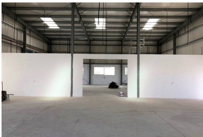
CLEAR-SPAN INTERNAL FLOOR
