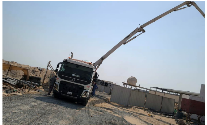
CONCRETE PLACEMENT BY BOOM PUMP
